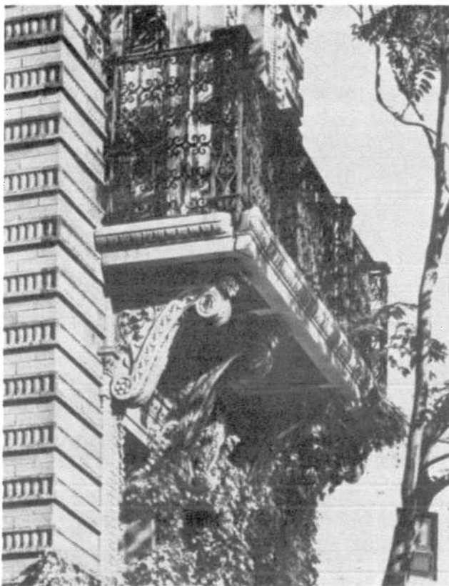
The terra-cotta quoins and window frames are seen here near the small balcony on the east side of the house. (Alan Hess, photographer)
